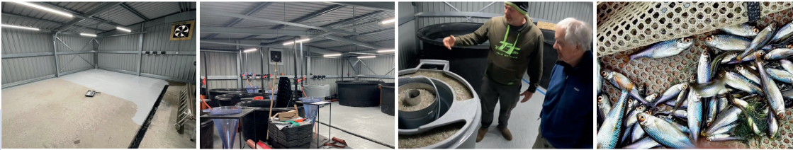
From an empty plot to the first fully functioning coarse fish hatchery on the Kennet
