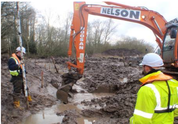
The new channel under construction
